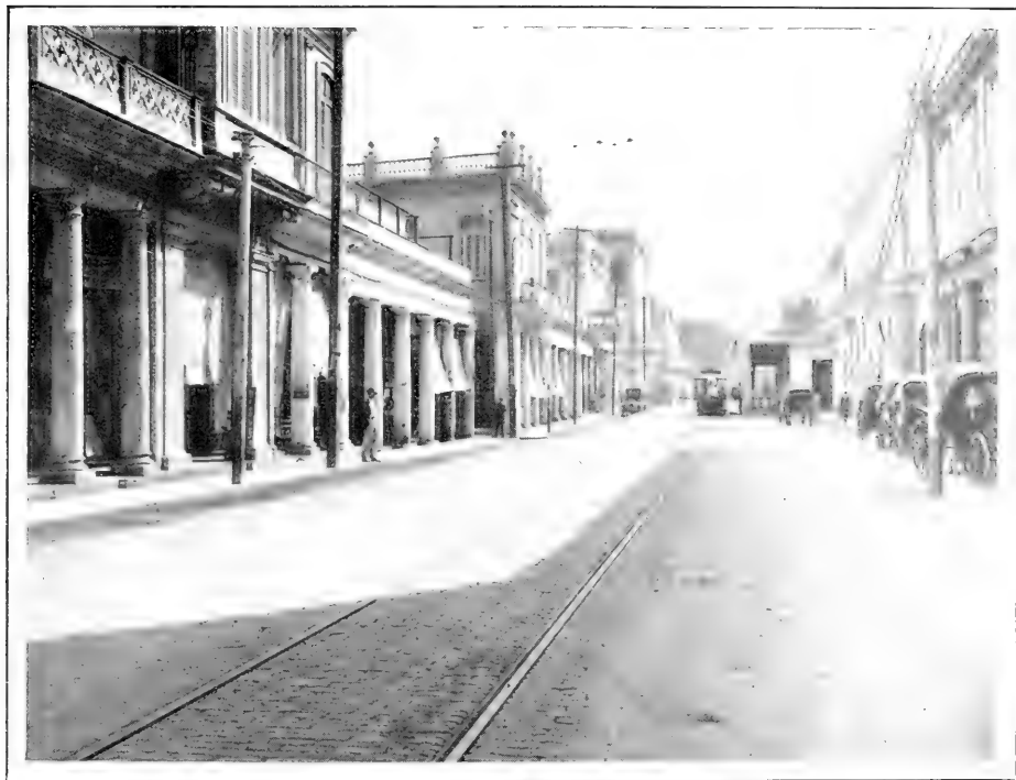
New Pavement Havana Streets.
